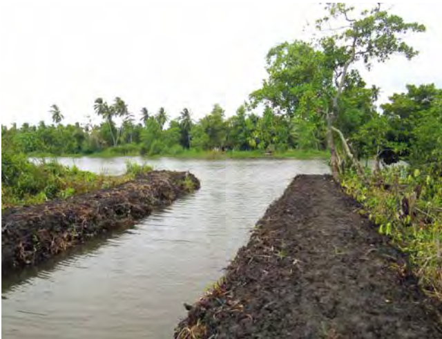
Left: Rehabilitated drainage channel.
